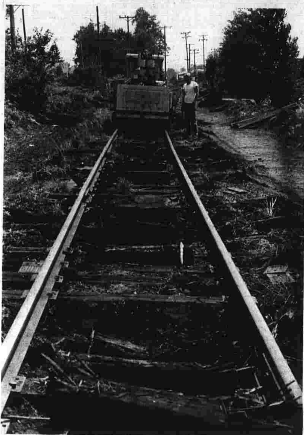
Railroad tracks undergo repairs
